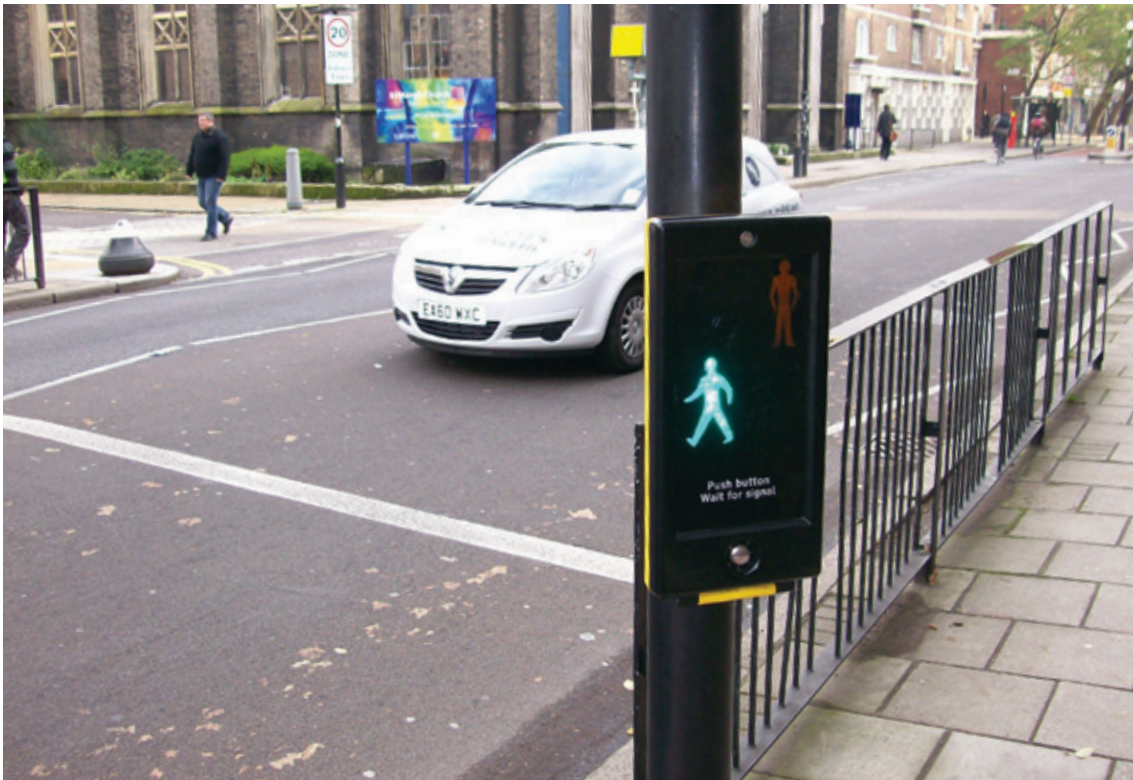
Figure 3: Puffin Crossing with nearside sign showing red or green
