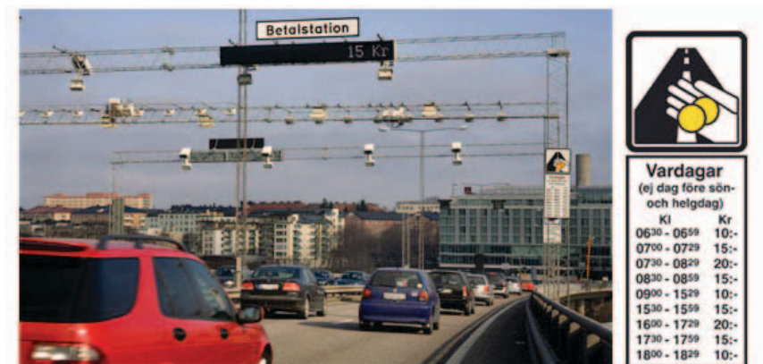
Figure 14: The Stockholm congestion charging scheme – gantries
