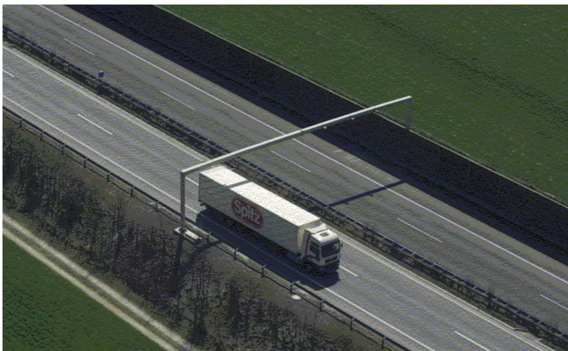
Figure 25: A charging point in the Austrian lorry charging scheme
